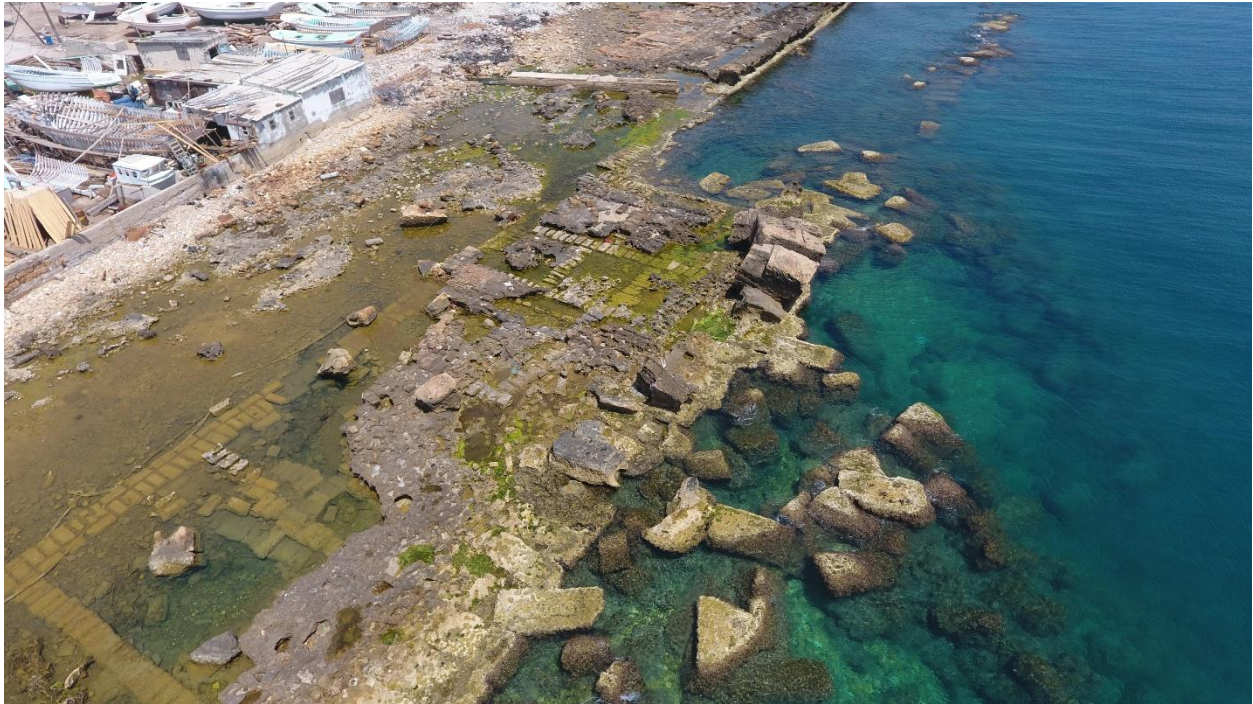
[FIGURE 8]: Aerial view of the southern side of Arwad island showing the submerged archaeological remains and the submerged coastal fortification wall © Taken by the researcher
