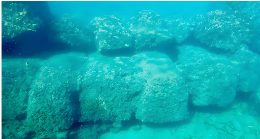
[FIGURE 6]: A submerged fortification wall at the south-east corner of Arwad island.
