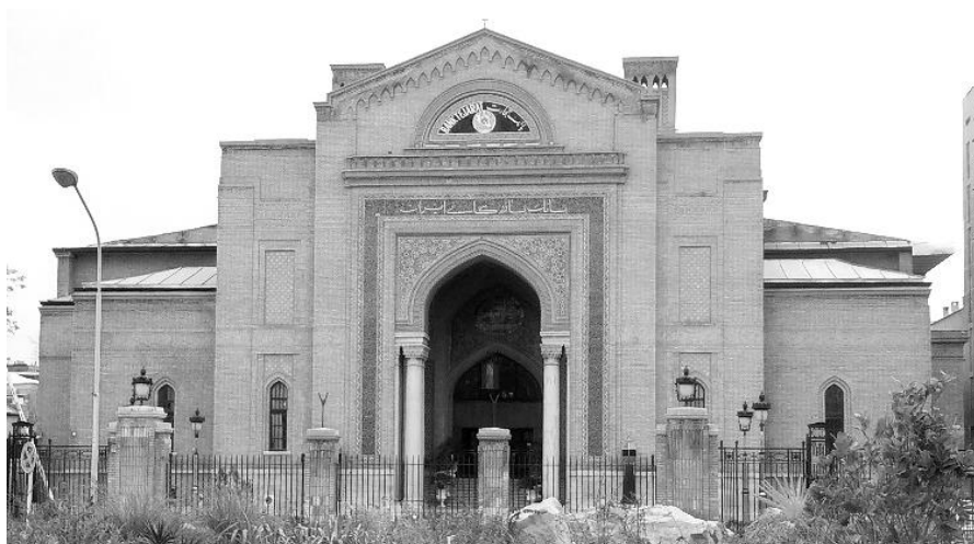
[FIGURE 13]: Former Imperial Bank of Persia building, east side of Tūphāneh Square. @Taken by the researchers.
