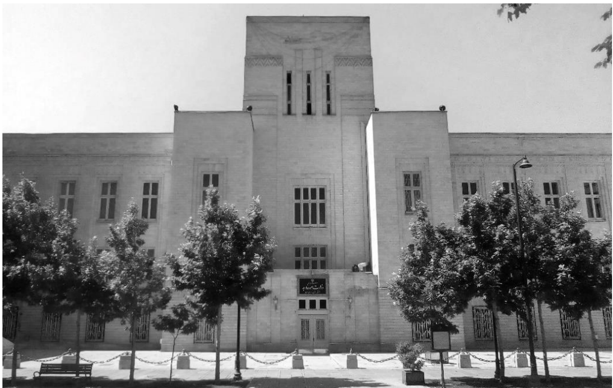
[FIGURE 17]: Ministry of Foreign Affairs Building N° 1, Tehran, @Taken by the researchers.
