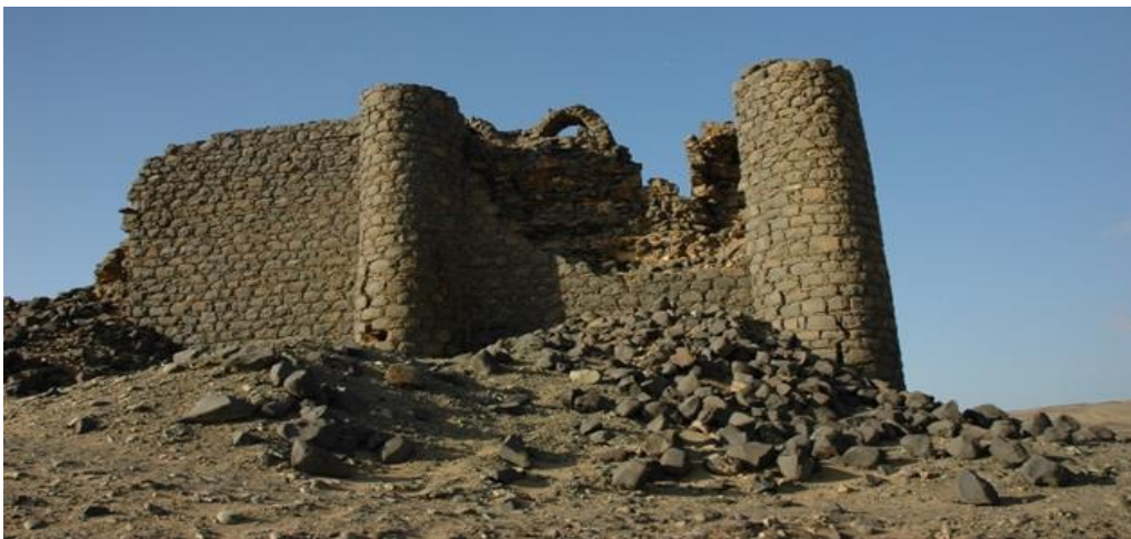
[FIGURE 4]. The southern façade of the Palace © Taken by authors
