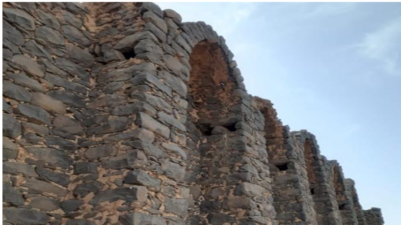
[FIGURE 8]. Openings of the wooden strings in the internal walls of the Palace © Taken by authors
