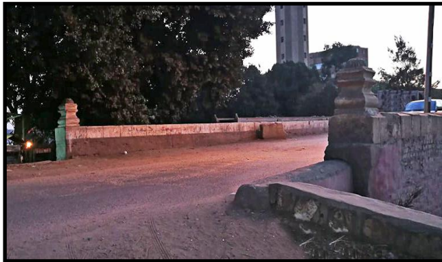
Plate No. 23: The eastern entrance of the upper road of the Bagouria barrage (Photographed by the researcher).
