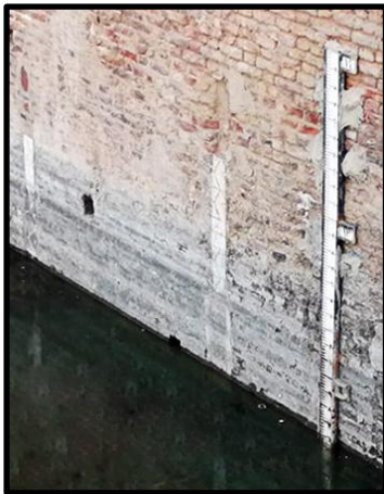
Plate No. 34: Three Nilometers located at the eastern wall behind the lock of the Bagouria barrage (Photographed by the researcher)
