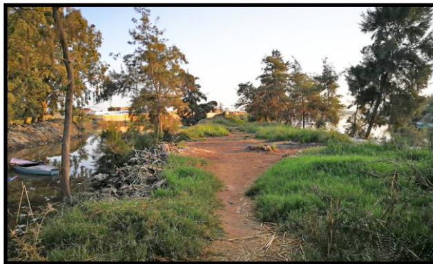
Plate No. 24: The embankment between the front entrance of the barrage and lock of the Bagouria canal (Photographed by the researcher)
