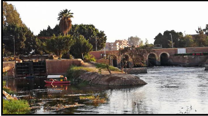
Plate No. 1: General view showing the barrage and the lock of the Bagouria (Photographed by the researcher).
