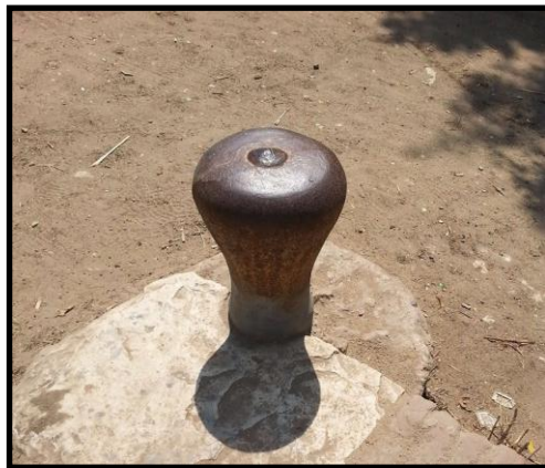
Plate No. 17: A metal peg used to tie the ropes of boats and ships at the Bagouria Lock. (Photographed by the researcher)
