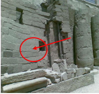
Fig. (6) Differential tendency on the walls of Luxor temple
