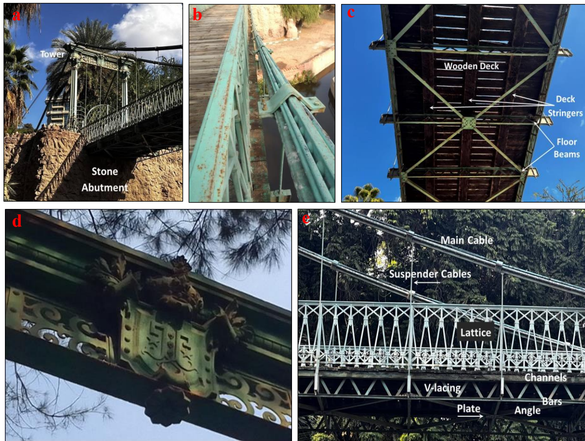
[FIGURES 4]: Parts of the bridge: A. The stone abutment and its tower; B. Main cables of the bridge; C. Deck stringers of the wooden deck; D. Eiffel's bridge plaque identifying the emblem of the Khedive Isma'îl; E. The main components of the superstructure part of the bridge © Photos taken by the authors
