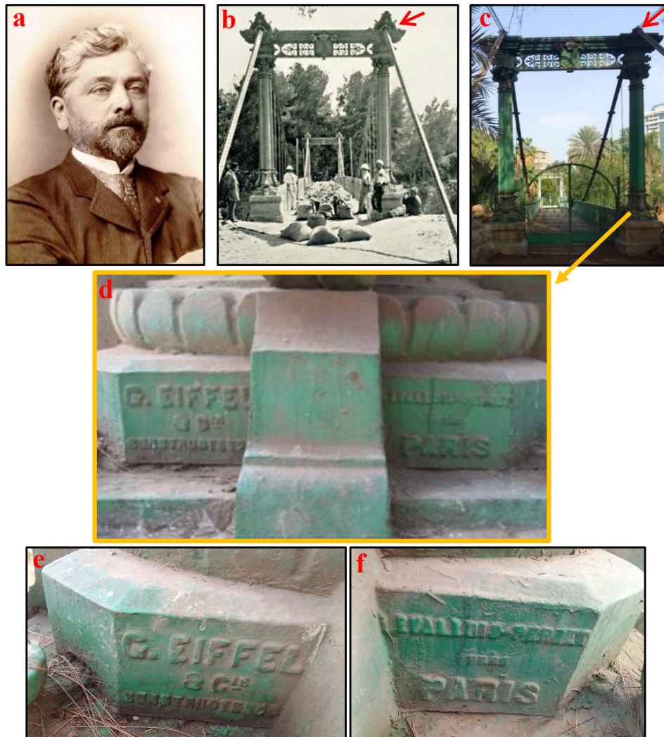
[FIGURES 2]: A. Gustave Eiffel, the designer and manufacturer of the bridge; B. Testing the Suspension Bridge in 1911 and the western entrance with a floral decoration from which the main cable emerges; C. A recent photo shows Eiffel's signature on one of the sides of the bridge's entrances without the floral decoration and a small gate was added; D. Detail of Gustave Eiffel and the company's construction marks on the bridge; E. Signature of Gustave Eiffel; F. Place of manufacturing the bridge © Photo taken by the authors
