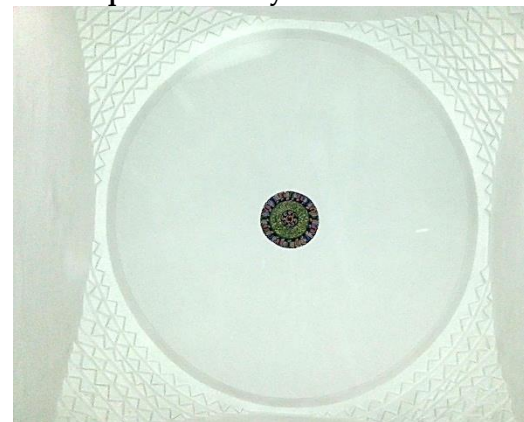
[FIGURE 18]: The transition zone of Dongsi domes © Photo taken by the researcher
