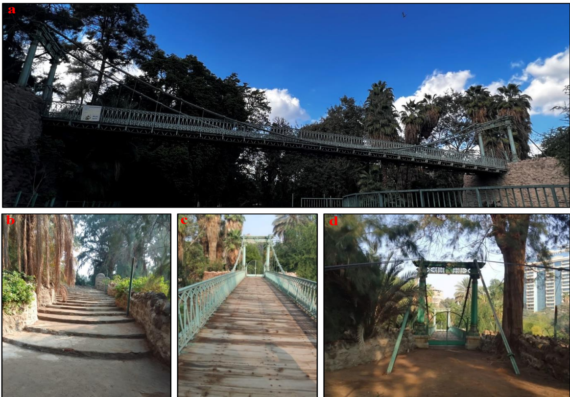
[FIGURES 3]: A. General view of the Eiffel Suspension Bridge; B. The ramp leading to the bridge at the stone abutment; C. The structure of the bridge; D. Its entrance from one end and fixing the main cable into an underground anchorage © Photos taken by the authors
