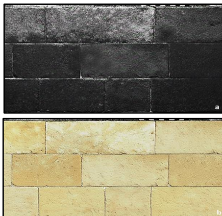
[FIGURES 16/A-B]: A. Shows the blackened limestone surface before treatment; B. The surface after chemical–biological treatment © Photo taken by the researchers
