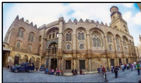
[FIGURE 14]: The Sultan Qalawun Complex with its façades affected by black crust, https://www.cairo.gov.eg/ar/pages/CairoInLines.aspx?CiLID=6 , accessed on (01/11/2025)
