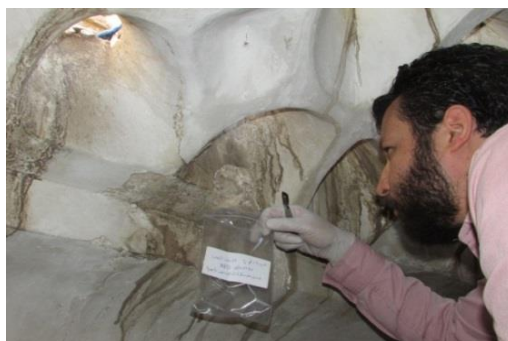
[FIGURE 10]: Shows taking 1A, 4D samples from bathroom ceiling stucco dome © Photo taken by MOHAMED ATYIA HAWASH
