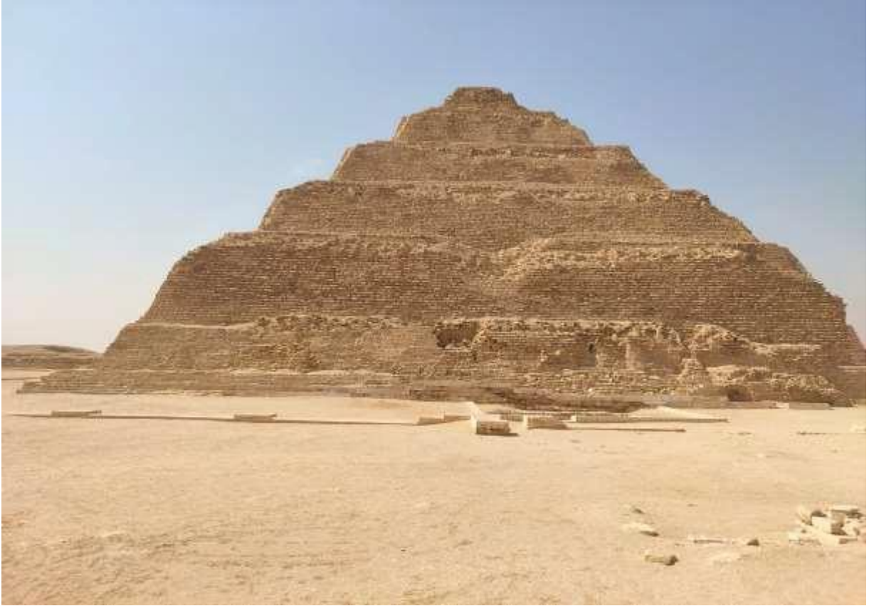
[FIGURE 3]: South façade ©credit by HAWASS 2006.
