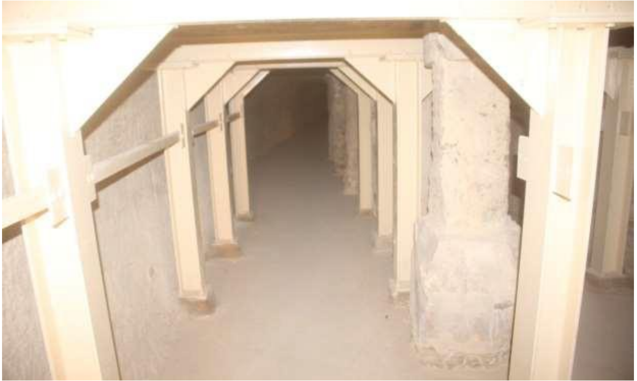
[FIGURE 5]: Restoration of the South entrance © credit by HAWASS 2018.
